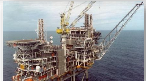
JASMINE PLATFORM 18.225 t platform DRAGADOS OFFSHORE
